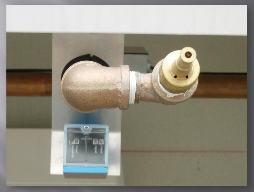
A sensor mounted beneath the nozzle will only allow a dock door to be sprayed IF a trailer is present, eliminating indiscriminate use of water.
