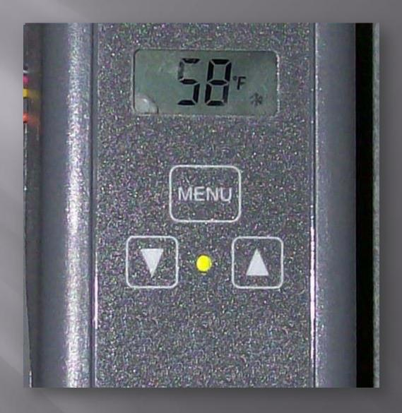
A thermostat wired into the control scheme ensures the system only operates when temperatures are hot enough to allow for evaporation – a feature designed to prevent unnecessary use of water.
