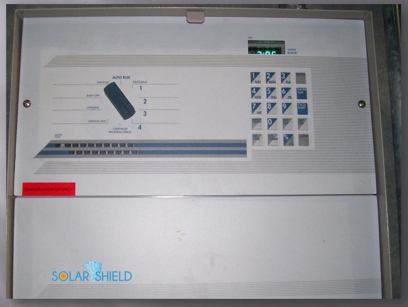
The entire truck spray system is hard wired to a programmable control box. The box groups dock doors together in "zones." This means multiple doors could be sprayed at a time, depending on water pressure.
