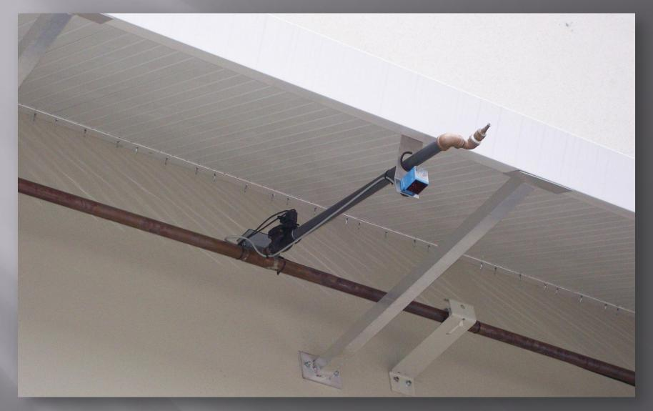
Each dock door is equipped with a spray nozzle assembly designed for maximum roof coverage and evaporative effect.
