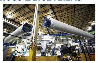
By placing 3" holes the length of the tubes, employees experience air movement without having to stand directly in front of a high velocity fan.
