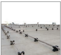
Evaporative Roof & Truck Cooling Roof spray system - Eliminate heat buildup at ceilings; Reduce inside temps
